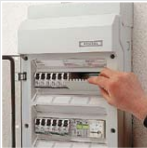
12 to 54 modules: attached blanking strips for DIN rail equipment openings
