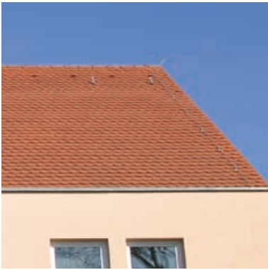
Figure 5.1.2.1 Air-termination system on a gable roof
