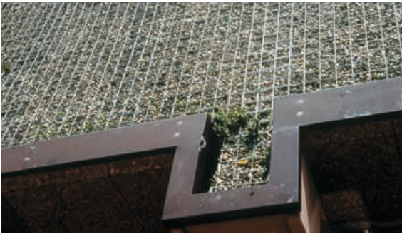
Figure 7.3.7a Galvanised reinforcement mats for shielding the building
