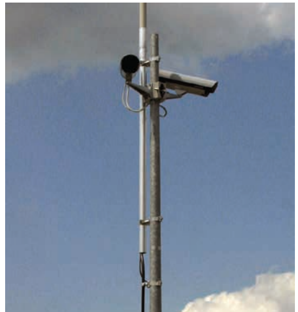
Figure 9.22.4 HVI Conductor installed at a pylon
