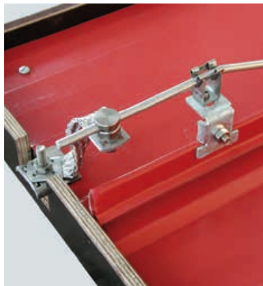
Figure 5.1.4.6 Sample construction on a standing seam roof
