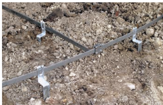
Figure 5.5.2.25 Spacer with cross unit
