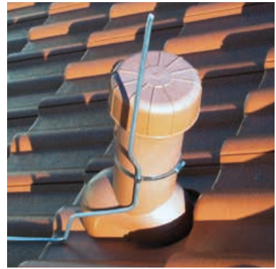
Figure 5.1.2.3 Additional air-termination system for vent pipes
