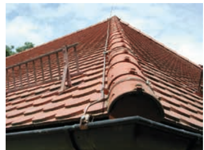
Figure 5.2.2.1.3 Air-termination system connected to the gutter
