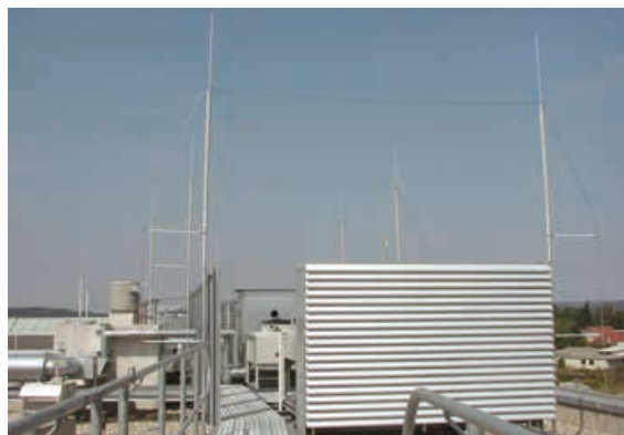
Figure 5.1.8.11 Isolated air-termination system with DEHNiso Combi
