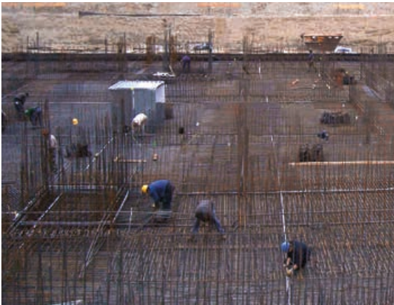
Figure 5.5.2.6 Meshed foundation earth electrode
