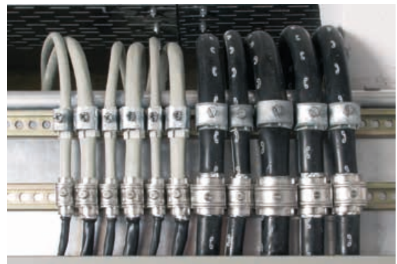
Figure 6.3.4 Lightning current carrying shield connection system (SAK)
