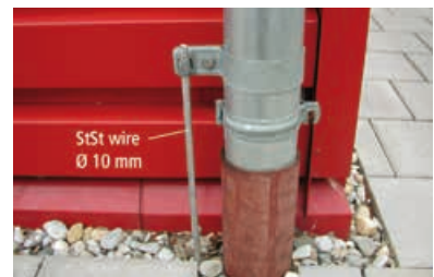
Figure 5.2.2.1.4 Earth connection of a downpipe
