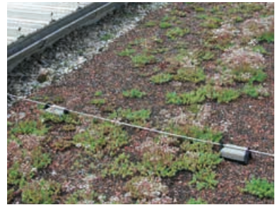
Figure 5.1.7.3 Conductor routing above the cover layer
