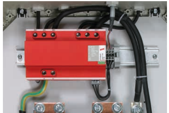
Figure 9.18.8 DEHNlimit PV 1000 V2 spark-gap-based type 1 combined arrester
