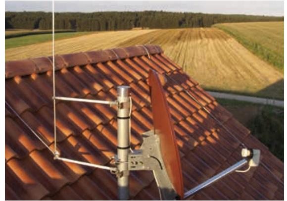
Figure 5.1.2.5 Antenna with air-termination rod and spacer
