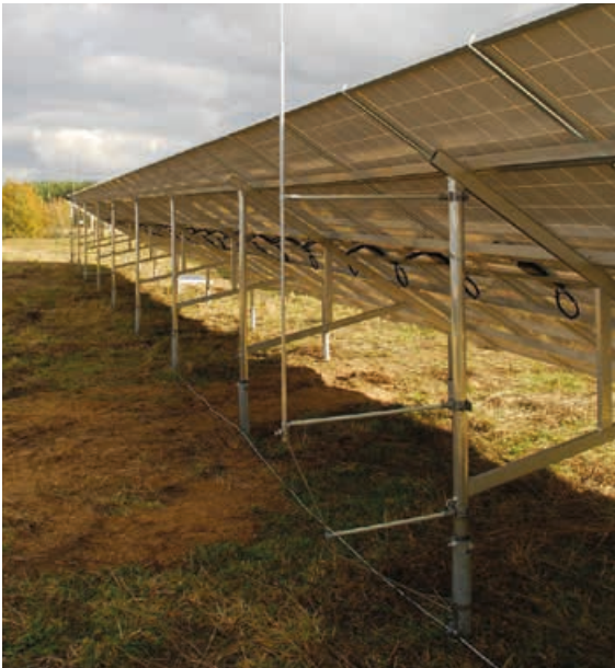
Figure 9.19.2 Lightning protection by means of DEHNiso spacers
