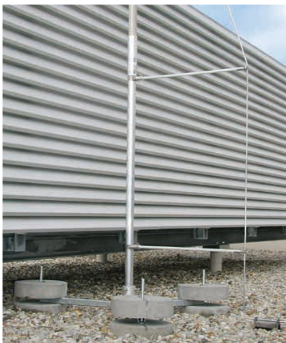
Figure 5.1.8.10 Tripod for isolated supporting tubes
