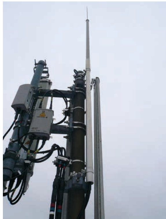
Figure 5.2.4.14 HVI Conductor installed on a radio tower
