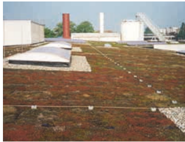
Figure 5.1.7.2 Air-termination system on a green roof
