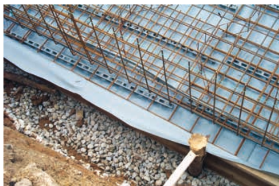
Figure 5.5.2.10 Membrane of foundation slabs
