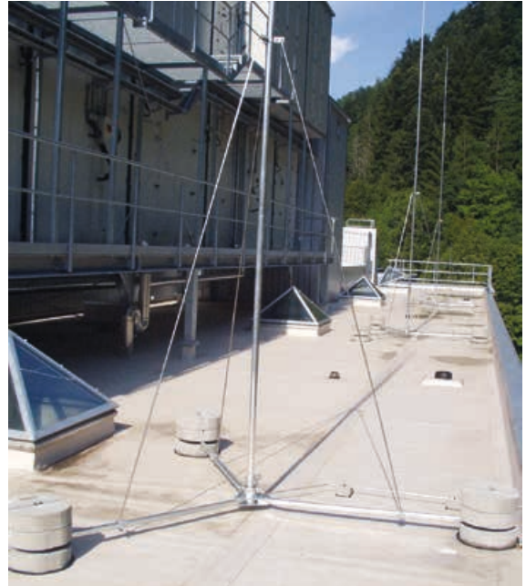
Figure 5.1.8.7 Isolated air-termination system for roof-mounted structures
