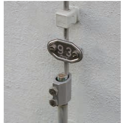
Figure 5.2.2.3.1 Test joint with number plate
