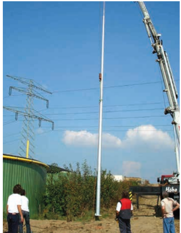
Figure 5.1.8.8 Installation of a telescopic lightning protection mast
