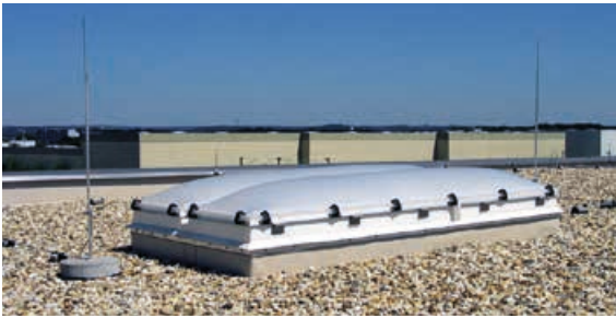
Figure 5.1.1.17 Protection of small-sized roof-mounted structures against direct lightning strikes by means of air-termination rods
