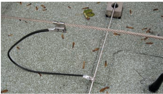
Figure 5.1.12.4 Flat-roofed structure – Detailed view
